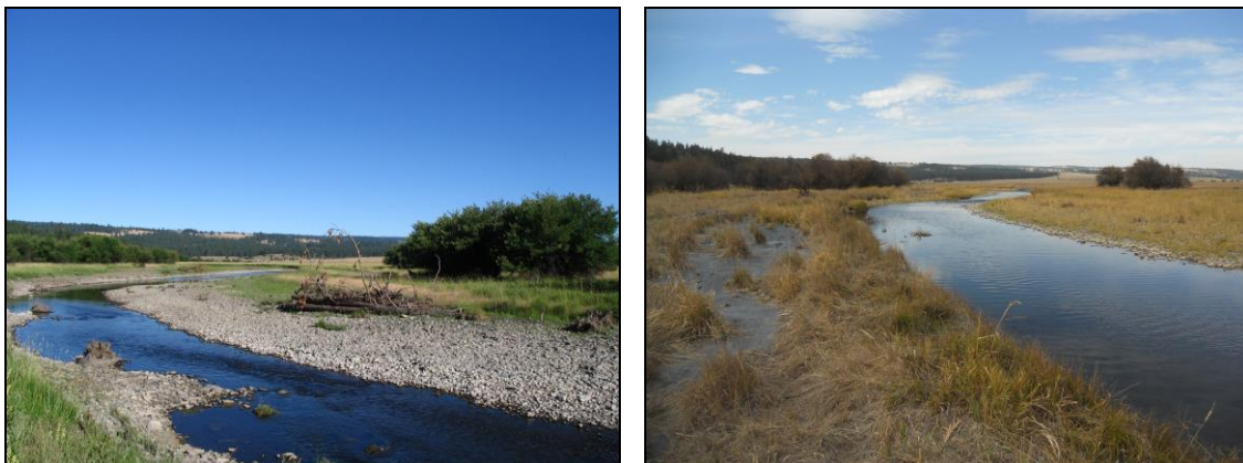
Figure 8. Photo point collected for the Lower Camas Creek site (right) 2007 a year after levee removal looking downstream with the lowest two J-hook structures visible. During 2015 (left) looking downstream from the middle of the reach where the lowest two J-hook structures is visible.
